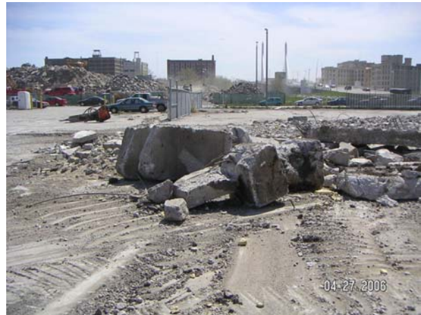
Removed concrete foundations; aggregate storage for crushing in background
