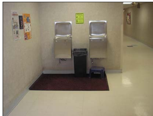
Reused drinking fountains replace leaking units St. Paul school
