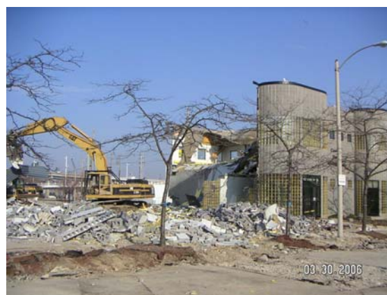
Demolition of Traser Yards Headquarters building
