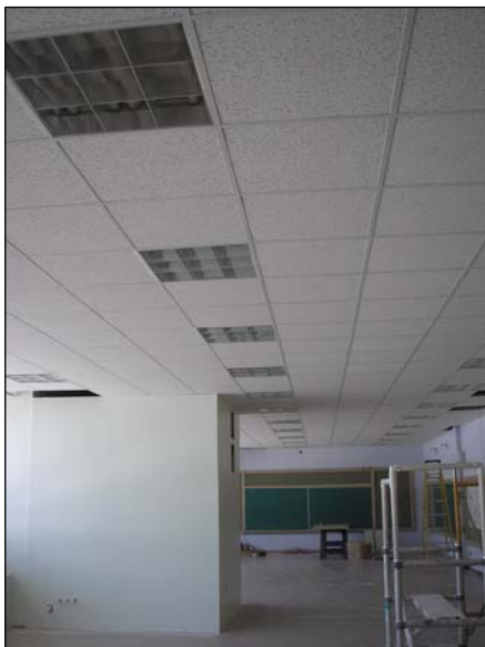
Re-lamped 2 x 2 light fixtures at St. Paul school
